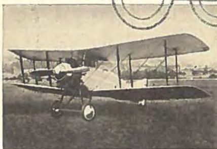
1921 - THE GLOSTER MARS, ancestor of all Gloster aircraft. The Mars I won the Aerial Derby three times. The Mars VI, illustrated above, was a fighter fitted with an Armstrong Siddeley 'Jaguar' engine.
